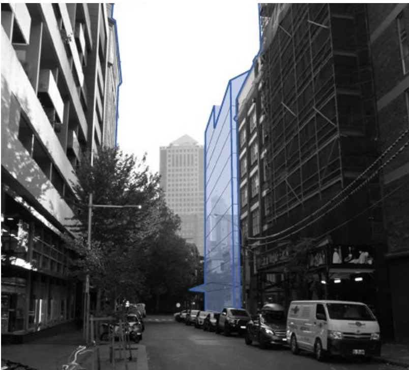
Figure 21. Proposed building envelope – viewed from Reservoir Street facing west
