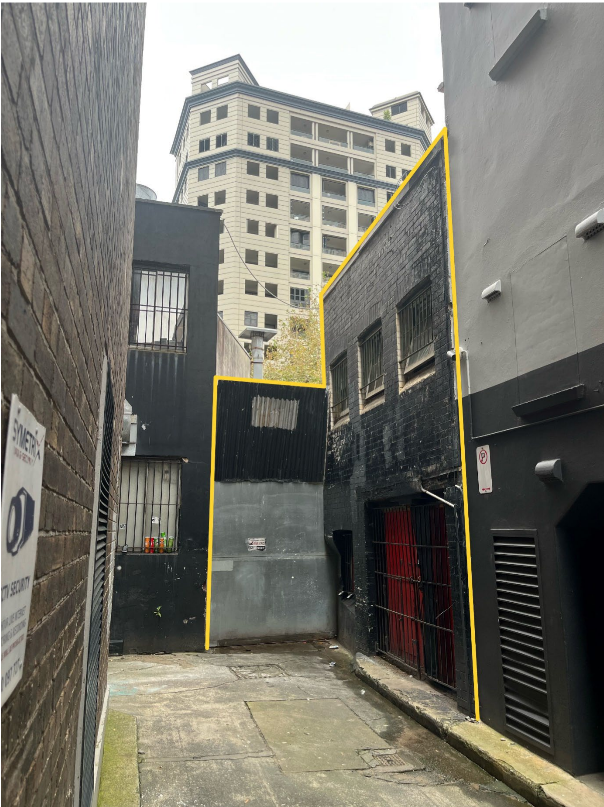
Figure 7. 232-240 Elizabeth Street, viewed from the north, outlined in yellow (access to Foster Lane)
